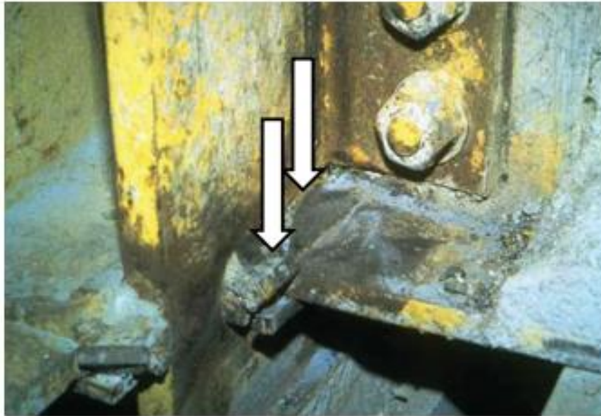
Fig. 6-2. Fracture of beam flange at CJP groove weld of beam flange to column flange. (Photo by Dave Norris)
